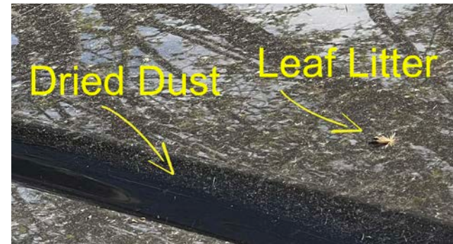
Flood to remove loose litter and moisten surface
