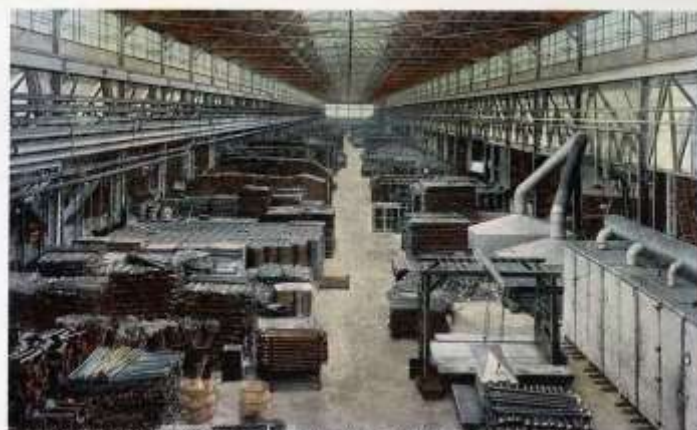
MAIN CRUMWAY, SHOWING STORAGE OF OVER $1,000,000 WORTH OF STOCK.
