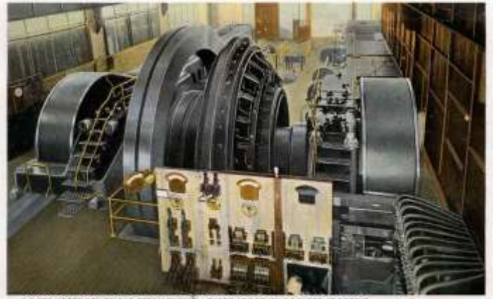
A 8,000 HORSE POWER GAS-STEAM ENGINE. THERE ARE SEVEN OF THESE AT FORD'S.
